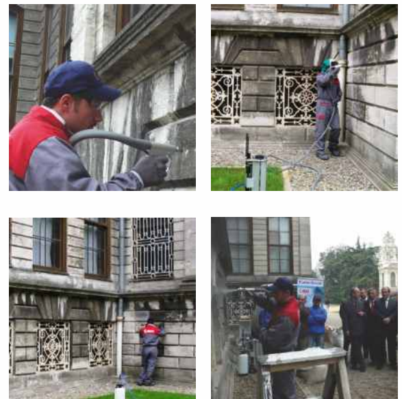
Dolmabahce Palace – Kufeki stone dry & micronised water and sodium carbonate cleaning.
