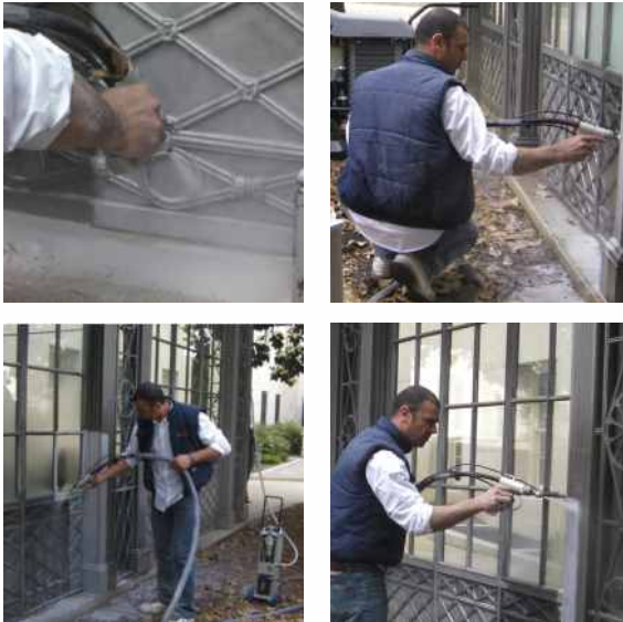
Cleaning of aluminum structures from particulate air pollution with sodium bicarbonate.
