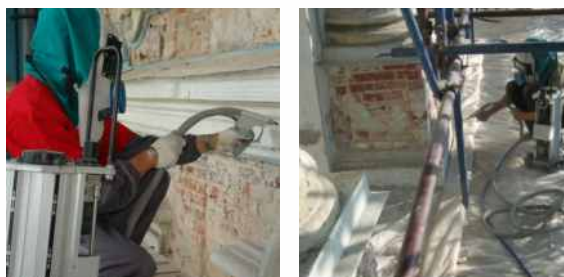
Catherine Palace (1717) – cleaning of persistent facade deposits with almandite.
