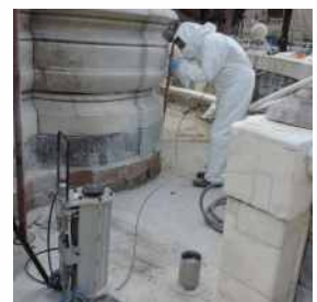
Fountain of Neptune (1595) – removal of lime deposits with calcium carbonate and water spray.
