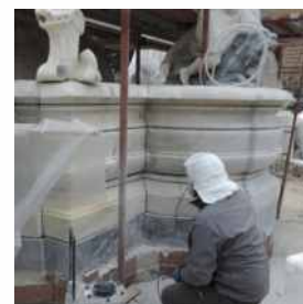
Fountain of Neptune (1595) – removal of lime deposits with calcium carbonate and water spray.
