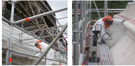
Eiffel Tower (XIX century d.C.) – cleaning of stone pillars with almandite 80 mesh.
