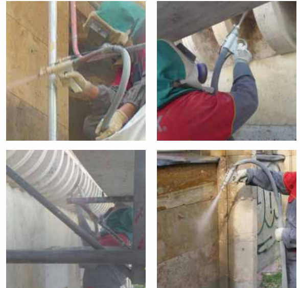
Post Office Building – cleaning of smog film with water vaporization.
