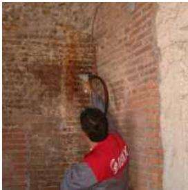
Imperial Forum of Trajan (1 century AD) – Cleaning of tuff stones and bricks, tuff bricks and mortar, travertine.
