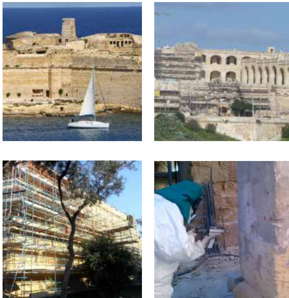
Walls XVI century – cleaning of delicate Maltese stone with sodium bicarbonate.
